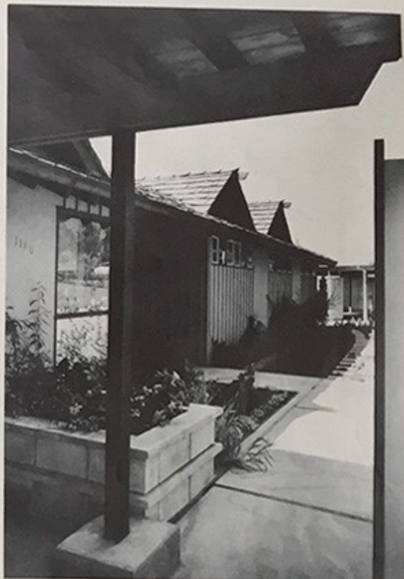
View from the carport shows the concrete entrance landing and flagstone path leading around shaded garden. Batten siding alternates with clear plywood panels to form decorative exterior treatment. Shake roof has no eaves troughs . . . dispersed drip falls on gravel drainage strip. Concrete block used for entrance planter repeats chimney detail.
